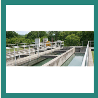
Water Treatment Plant Maintenance Services
