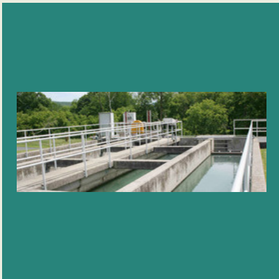
Water Plant Maintenance Contract Service
