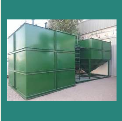
Package Sewage Treatment Plant
