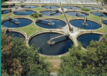
Industrial Wastewater Treatment Plants
