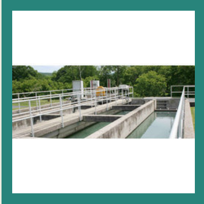
Water Treatment Plant Maintenance Services
