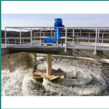
Modular Wastewater Treatment Plants
